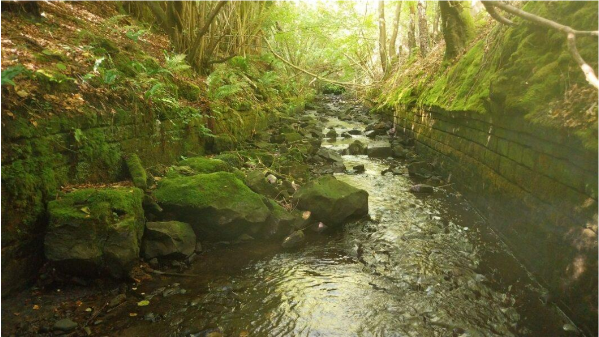
Figure 7 - Example of material deposition already occurring in some areas of the Blue Rock Trail due to wall collapse and other factors.
