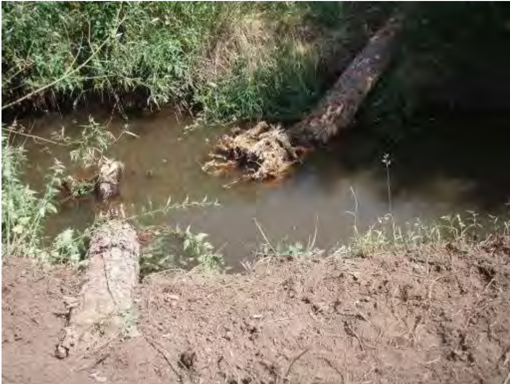
Photo 14 Root wads introduced to provide some in-channel structure and scour
