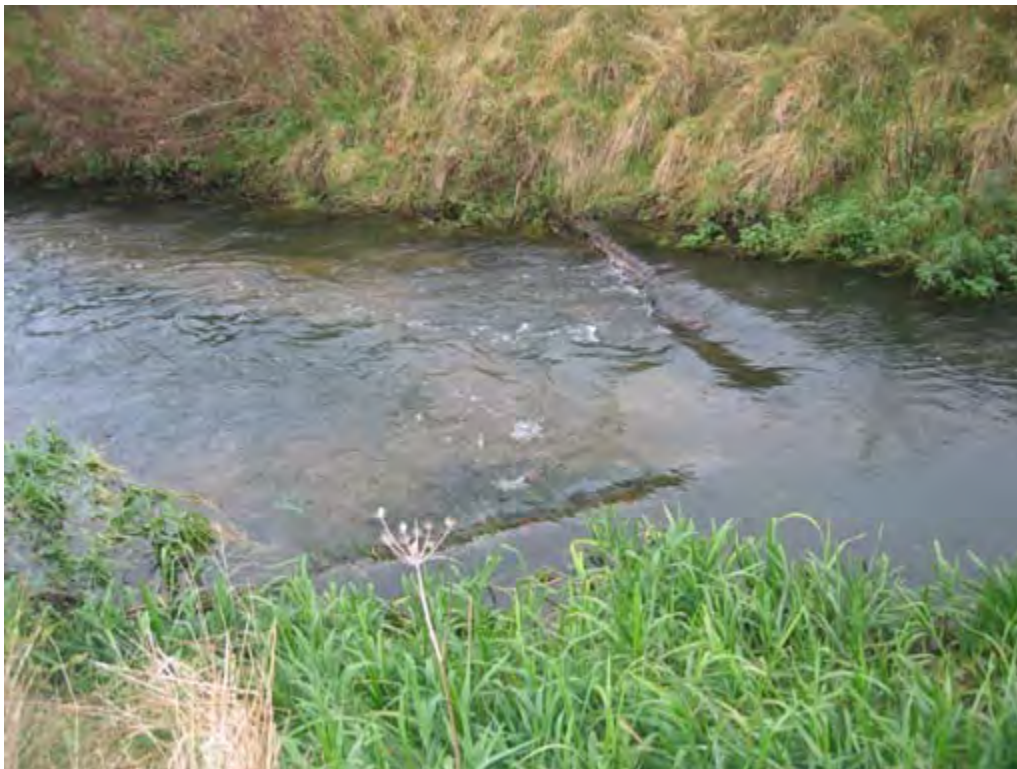
Photo 13 Paired log flow deflectors
